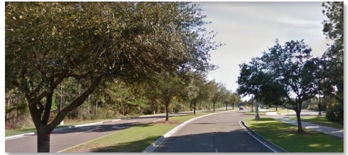
Figure 14: Trees within the right-of-way near the University of North Florida (Source: Google Maps)
