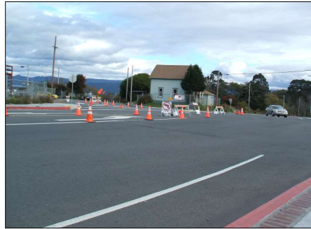
Signs, cones, and barricades were used to test the improvements before becoming permanent
