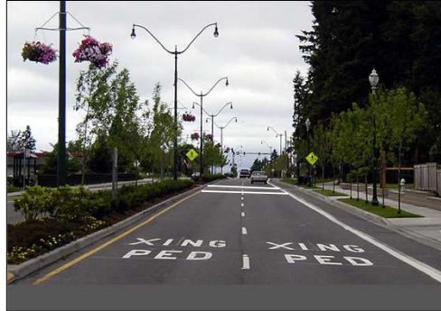
Mid-block pedestrian crossing
