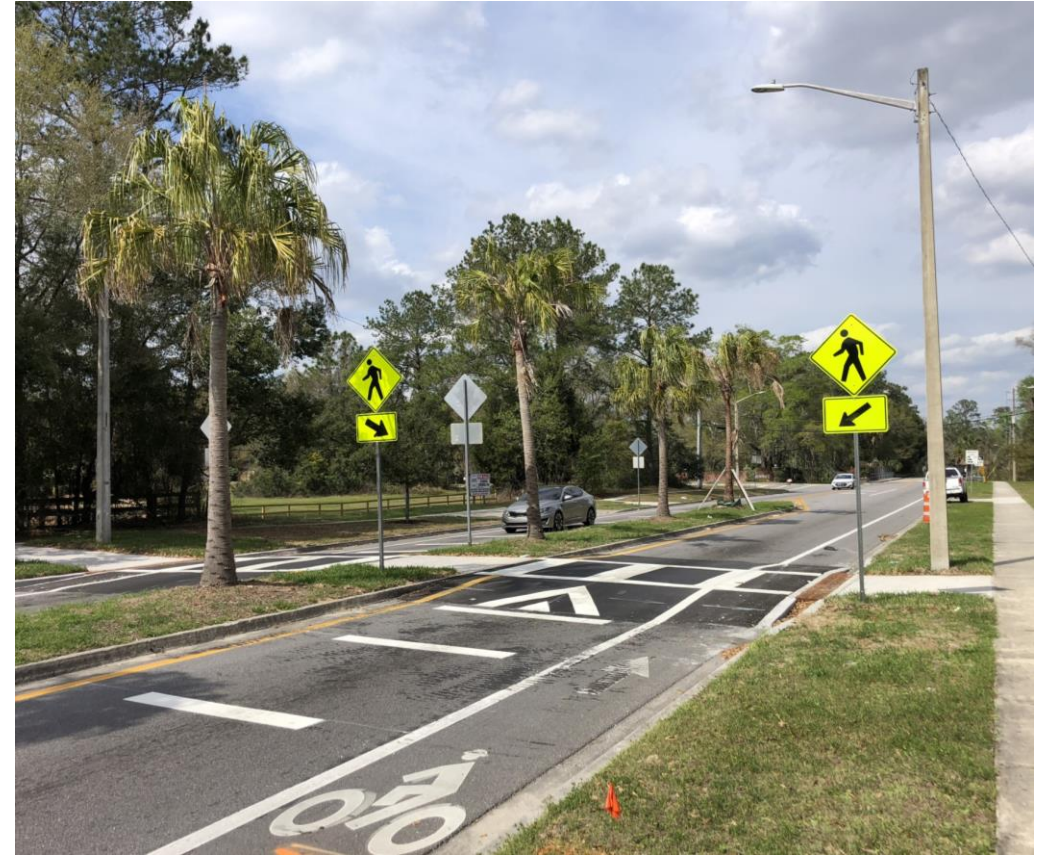
Raised median crossing with lighting & high-vis markings & signage on Harts Rd. in Jacksonville
