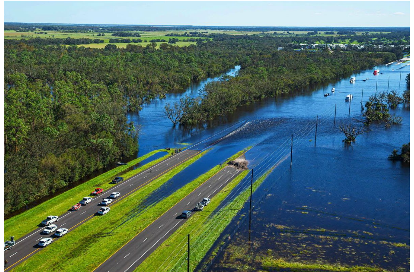
Image of highway disruption following Hurricane Ian Source: Geopix/Alamy Stock Photo
