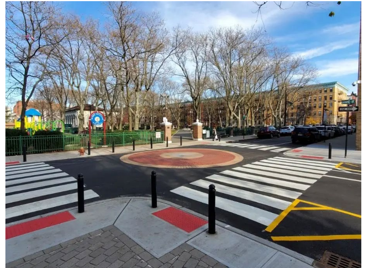
Narrower intersections with physical protections, like this one in Hoboken NJ, improve safety for all users
