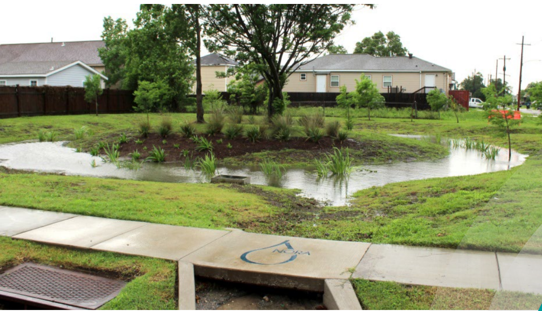
Reduced risk of flooding & damage
