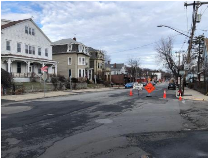
Intersection of Crescent Avenue at Broadway, Chelsea, MA
