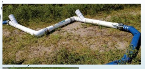
The link manifold is designed to eliminate the need for open dewatering ditches and allow for water treatment in-line with anionic polyacrylamide(PAM).
