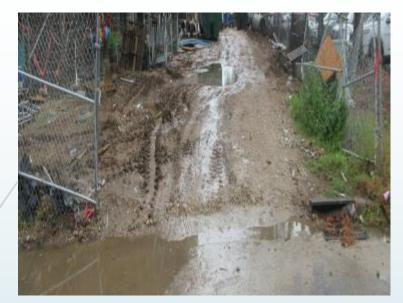
Stabilization to prevent track out is outlined with specificity in the manual. Track out is one of the largest contributors to unlawful discharges to stormwater. There are also reusable technologies available such as fods, rumble strips, etc.
