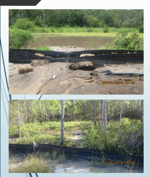
DEP Manual points out that black fabric does not protect against turbidity – recommends *double row* of silt fence and other turbidity controls
